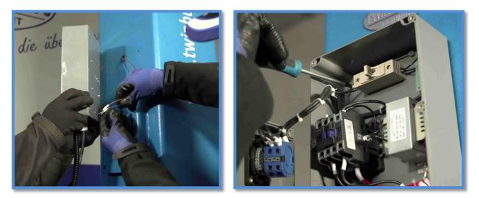
Now the motor cable can be connected.
